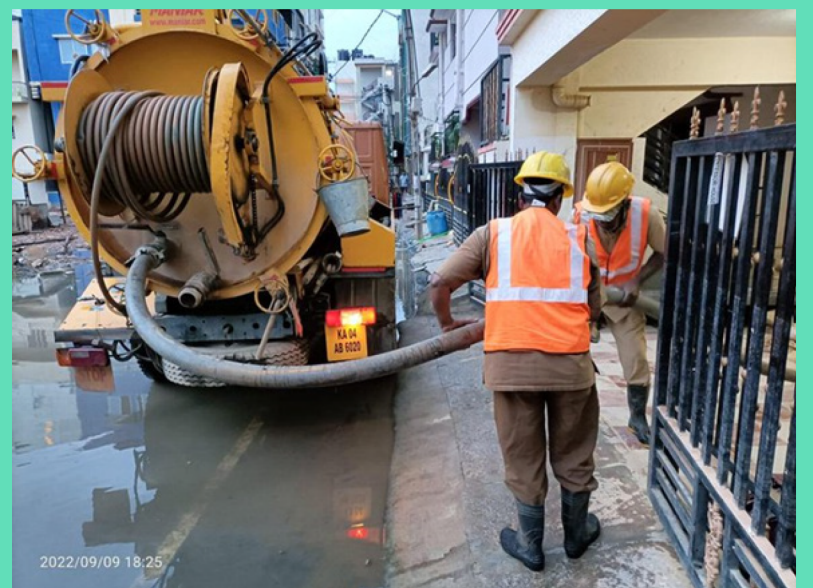
Using machines to clean toilets.
