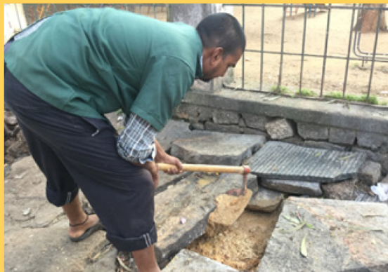
Cleaning septic tanks manually.
